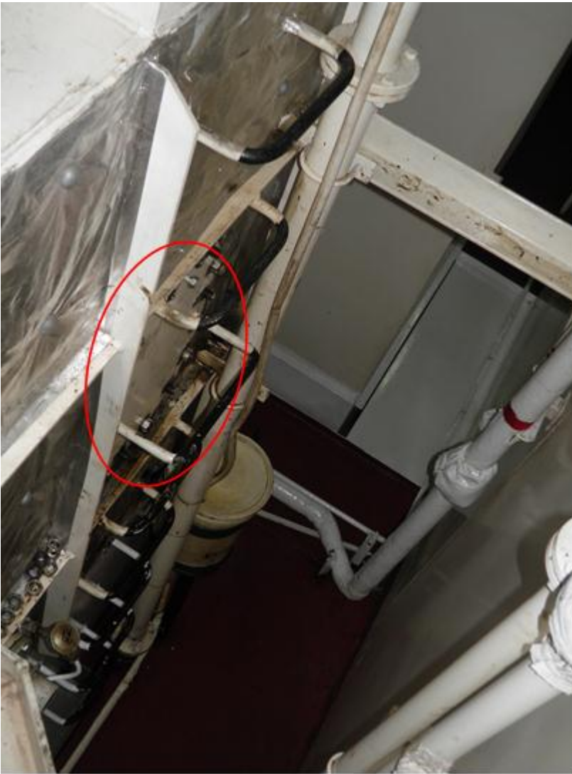
Figure 5: The manhole at the aft side of the tank almost one meter from the bulkhead and two meters from the floor.
